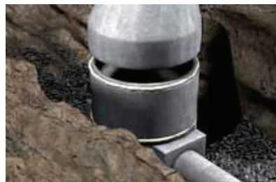
Sealing concrete manhole rings
